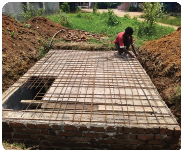
Construction of Roof Water Tank
