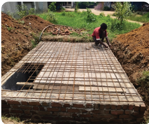
Construction of Roof Water Tank
